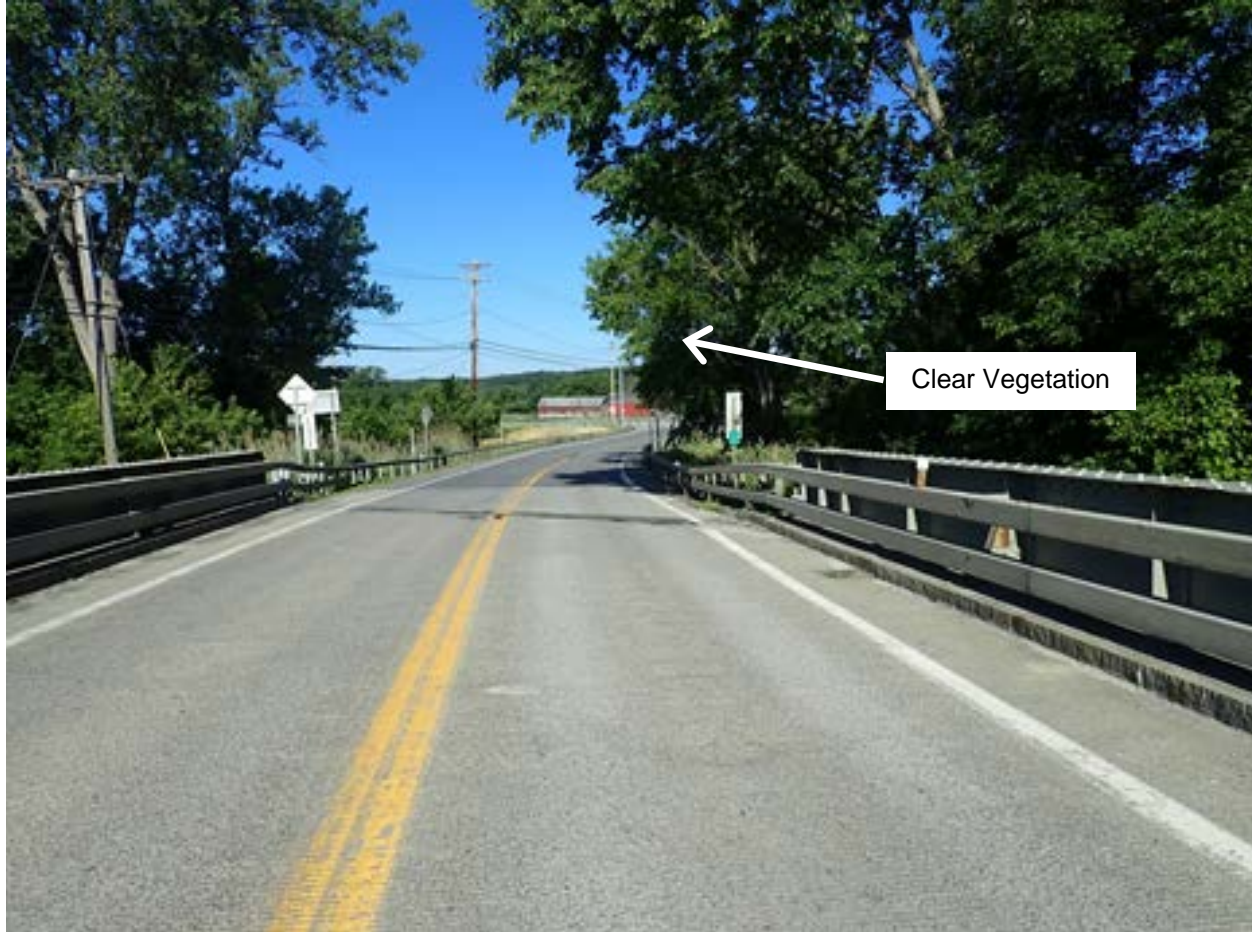
Photograph 1: Vegetation clearing to meet stopping sight distance guidelines.
