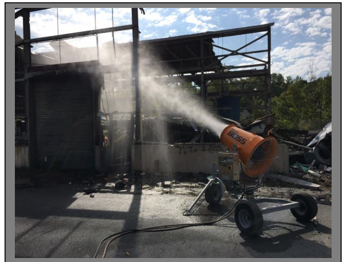
Example of equipment that may be used to wet building material during deconstruction.
