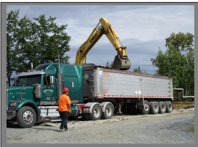
Example of loading truck for off-site disposal during deconstruction.
