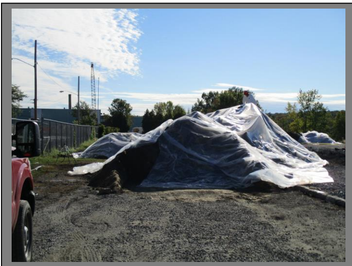
Example of covered stockpiles during deconstruction.
